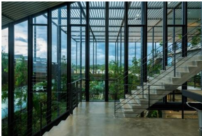
Gambar 5. Thermal and Airflow Variability pada Factory in the Forest Sumber: Design, 2017
