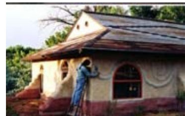
Gambar 5. The Allison Kennedy House di Utah, dengan dinding lurus Sumber: http://www.earthbagbuilding.com/projects/kennedyhouse.htm
