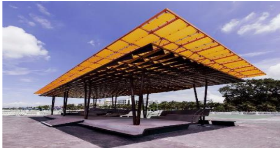
Gambar 3. The Flow , Chonburi Sumber : departmentofarchitecture.co.th
